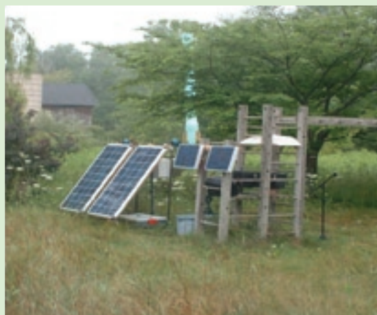
Figure 2. Field monitoring equipment
