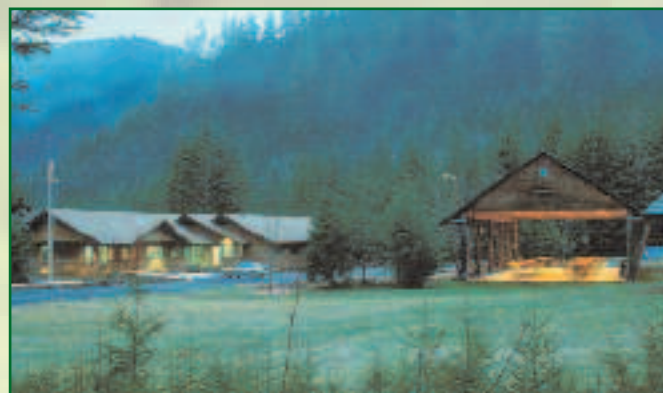
The Andrews Forest headquarters includes labs, offices, conference facilities, and lodging to support the field-oriented research program.
