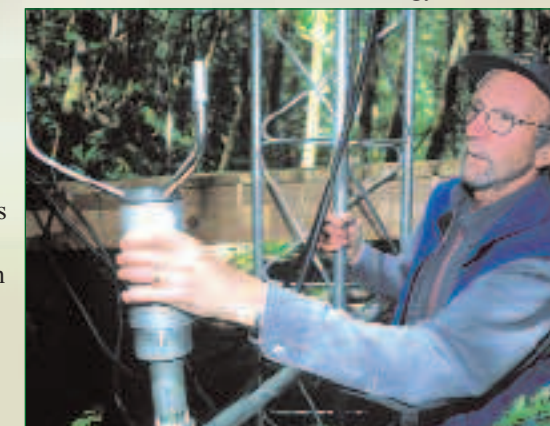
Installing a 2-dimensional anemometer to measure airflow patterns in the airshed of Watershed 1. Photo by Thomas Iraci
