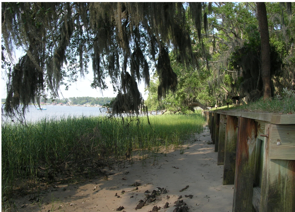
Figure 1. An intertidal bulkhead at the Skidaway Institution of Oceanography as an example of the shore parallel armoring structures focused on by the working group.
